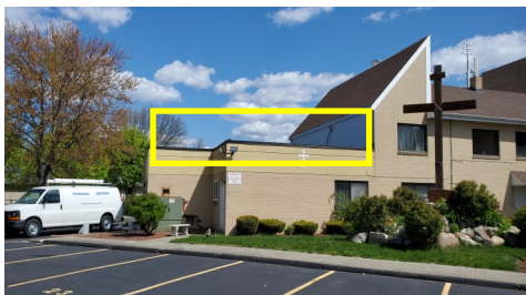
Rubber Roof (Rectory): $7,800.00
