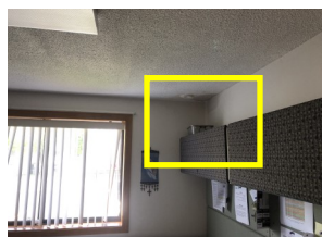
Rectory, Office, Kitchen & Garage Leak Damage Repair:
